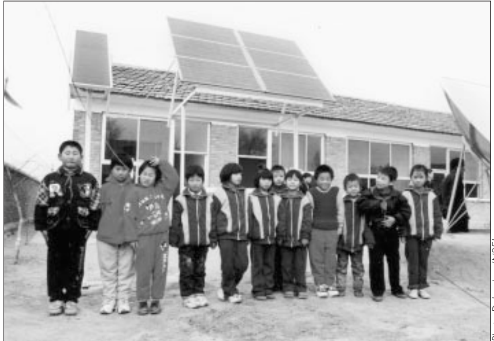
A PV-powered school in Beijing.
